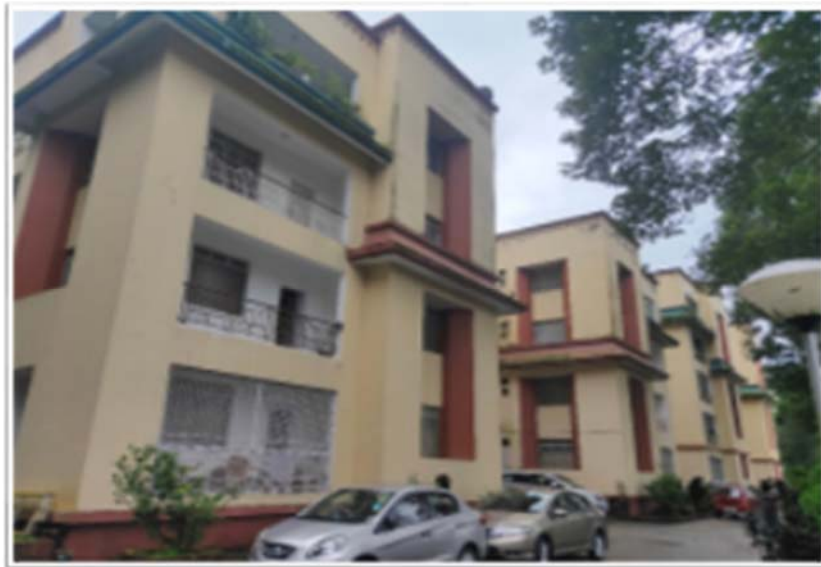
Staff housing at Medical Campus
