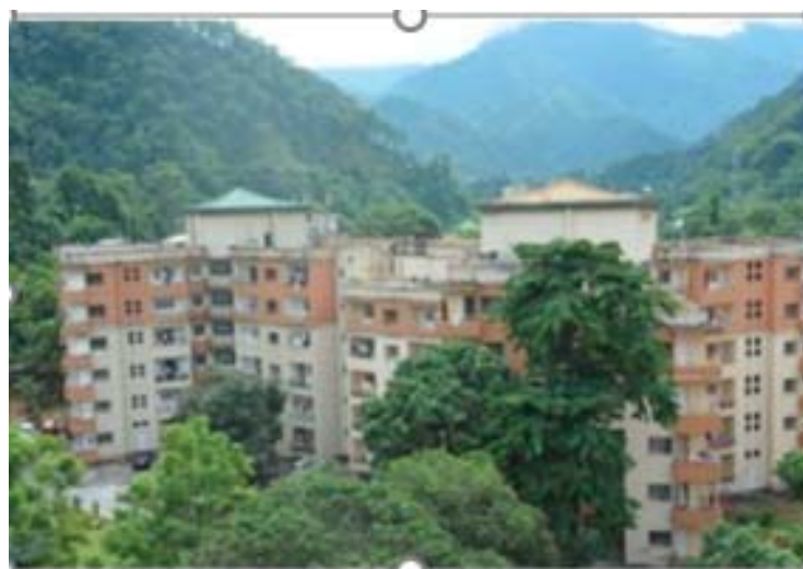
Staff housing at Engineering Campus
