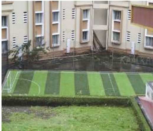
Well ventilated building structure
