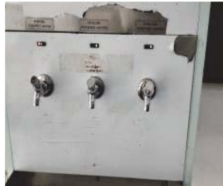
Push taps installed in water coolers
