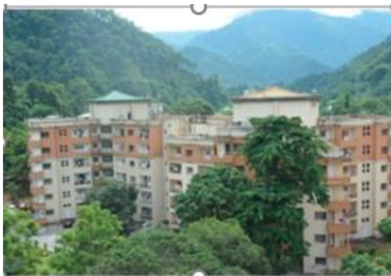
Staff housing at Engineering Campus
